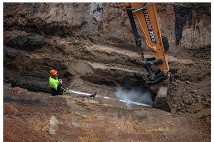
Culvert replacement works, Black Snake Creek Road July 2020
