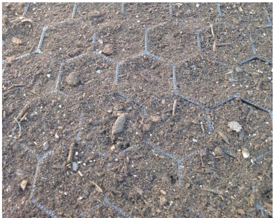
Geocell matting retaining soil
