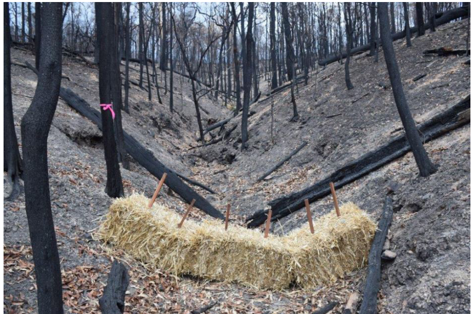
Strawbale systems for erosion control post fire
