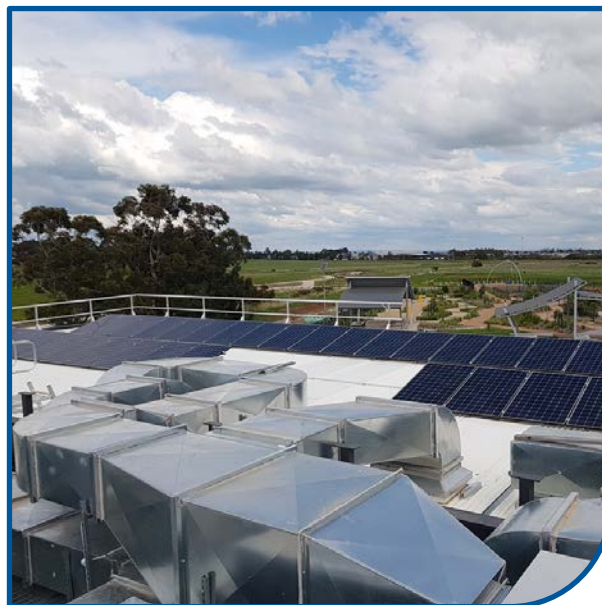
Photo: Solar electricity system and thermally reflective roof
