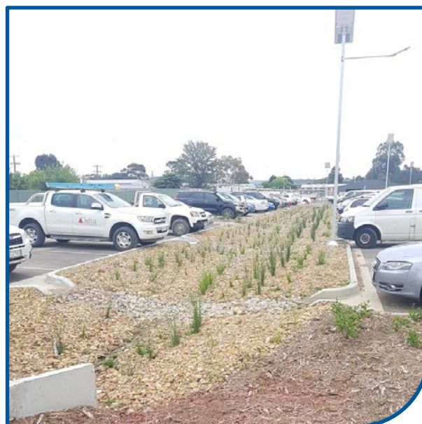
Photos: (L-R) Weather station. Car park with vegetated swale drains and independent solar lighting
