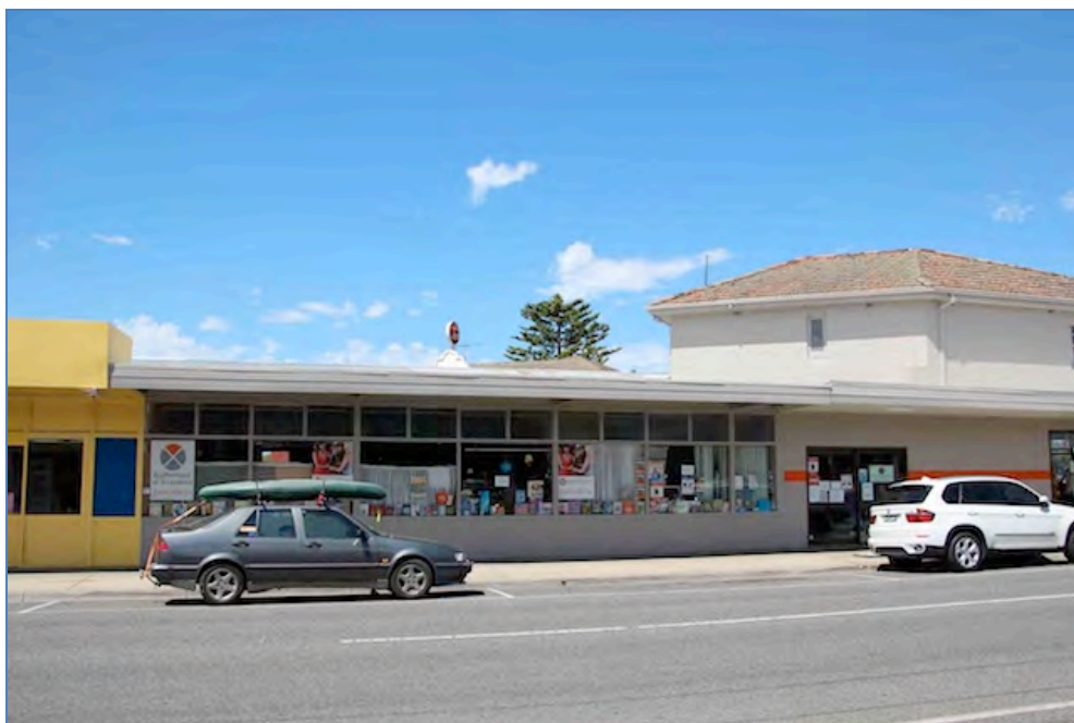
No.1-7 Station Street, Station Street facade
