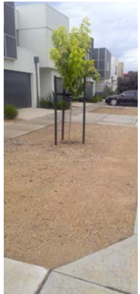
Permeable surface installed.
