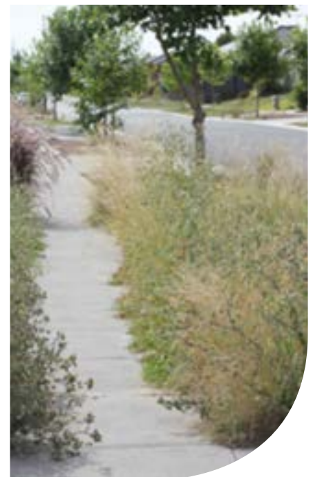
Nature strip is overgrown with weeds, exceeds the 300mm limit for grass and is encroaching on the footpath.
