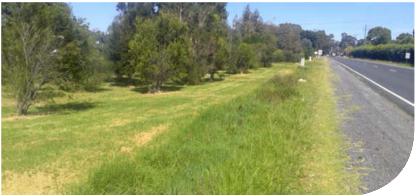
VicRoad arterial road.
