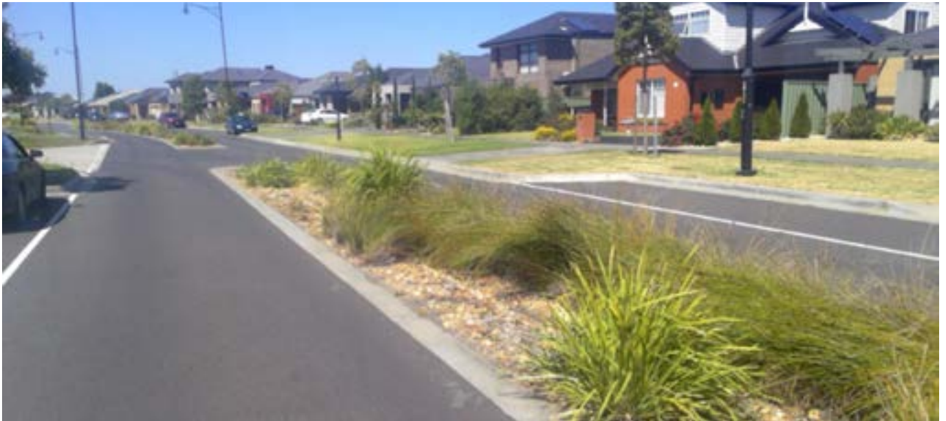
Water Sensitive Urban Design (WSUD) installation.
