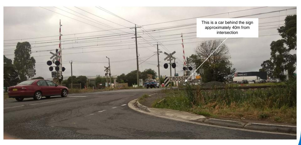
Sight line to south at 3m back from hold line at driver's eye height Total sight line is approximately 30m which is sub-standard. It is not possible to relocate the level crossing signs
