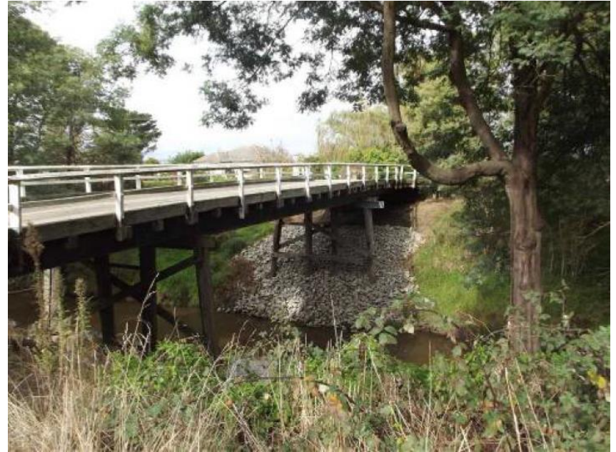
Looking at west side of Little Rd bridge
