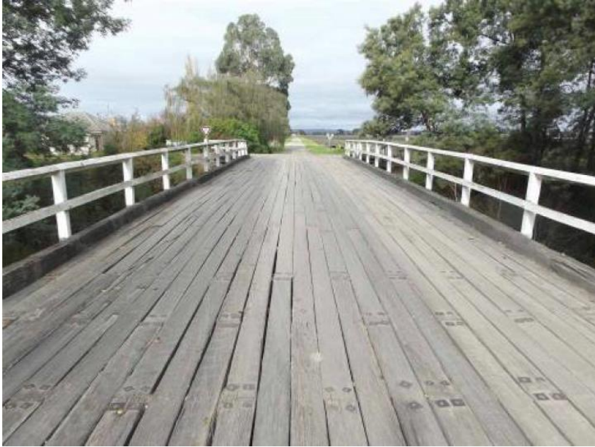
Looking south along Little Rd bridge
